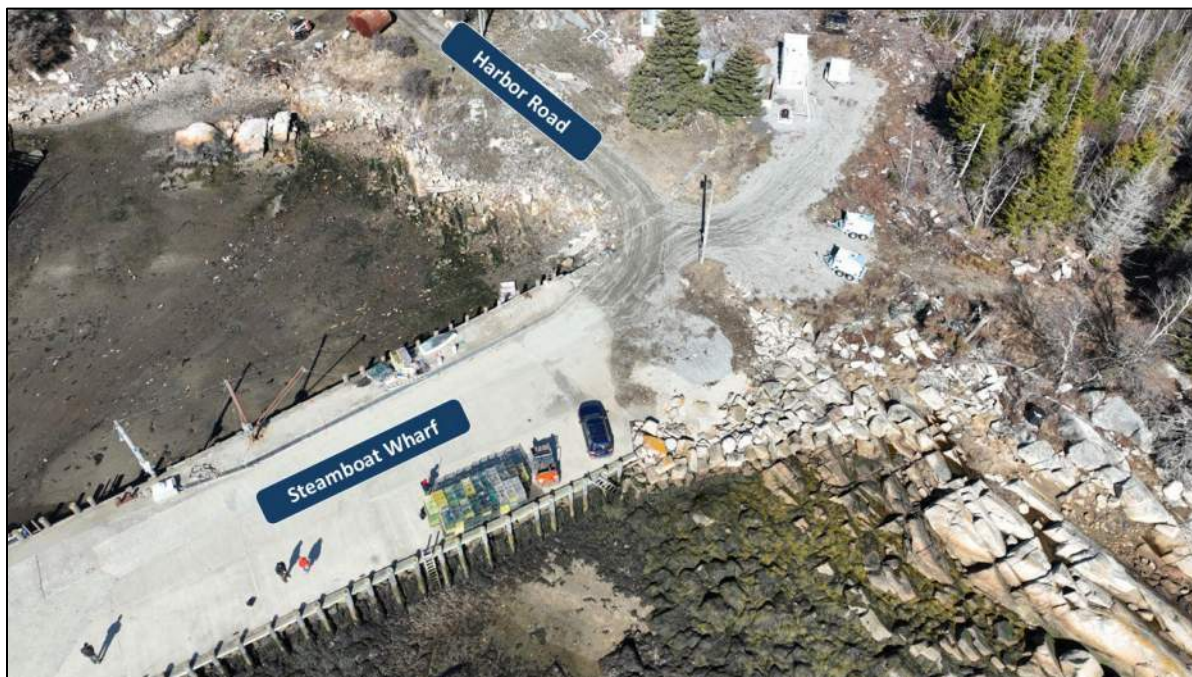
Figure 5-6. Aerial View of connection between Harbor Road and Steamboat Wharf
