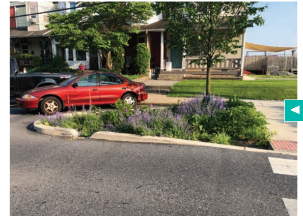
Crosswalk with stormwater bump-out in Lancaster City, PA.
