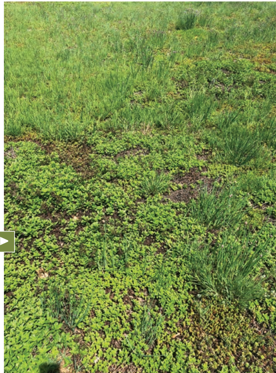
Typical green roof vegetation.
