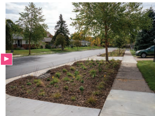
Tree trenches in Hoyer Heights, Minneapolis. (Photo credit- "Hoyer Heights Tree Trenches" by Mississippi WMO is licensed under CC BY-NC 2.0).
