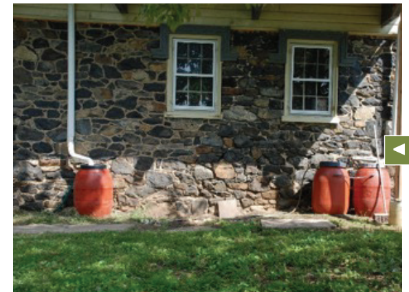
Typical rain barrel downspout connection, private residence.
