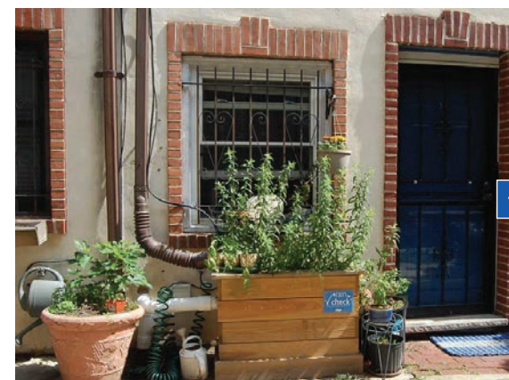
Residential downspout planter installed through the Philadelphia Water Department's Rain Check program. (Photo credit- "Downspout Planter" by Home Science is licensed under CC BY-SA 2.0).
