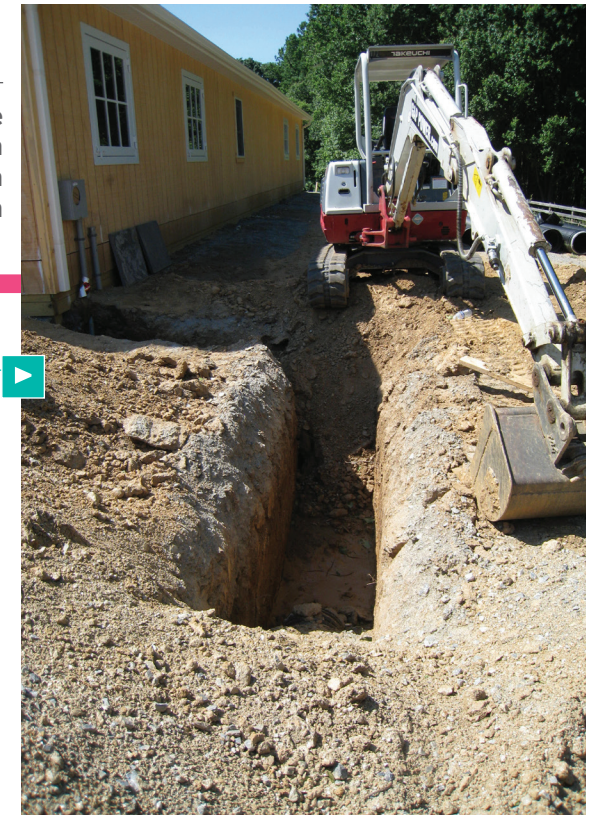
Excavation of hookup to underground infiltration system in Coatesville, PA.
