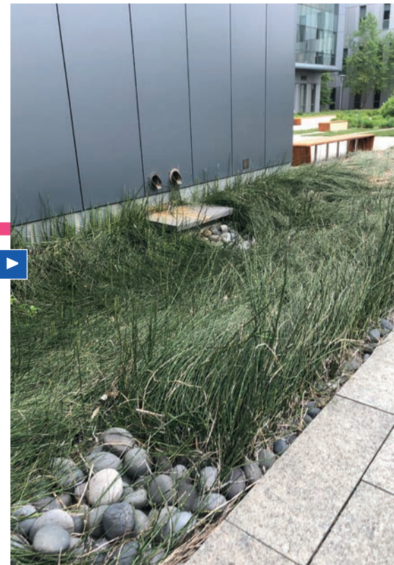
Large downspout planter at University of Delaware, Newark, DE.
