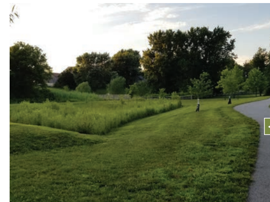
Bioretention basin in Unionville Community Park, East Marlborough Township, PA.
