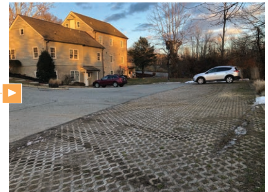
Pervious paver parking spaces at Chadds Ford, Chadds Ford Township, PA.
