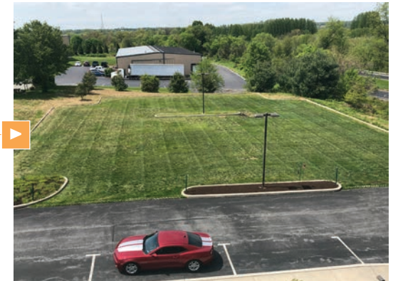
Pervious overflow grassed parking area at Dansko Company store and outlet, Penn Township, PA.
