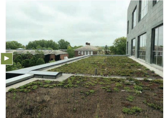
Green roof at University of Delaware, Newark, DE.
