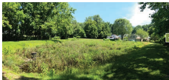
Residential bioretention basin in Westtown Township, PA.
