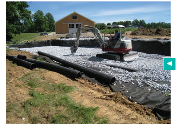
Installation of an underground infiltration system in Coatesville, PA.
