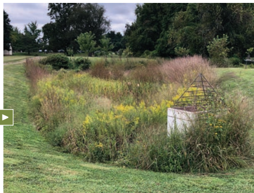
Bioretention basin at Hillendale Elementary School, Pennsbury Township, PA.
