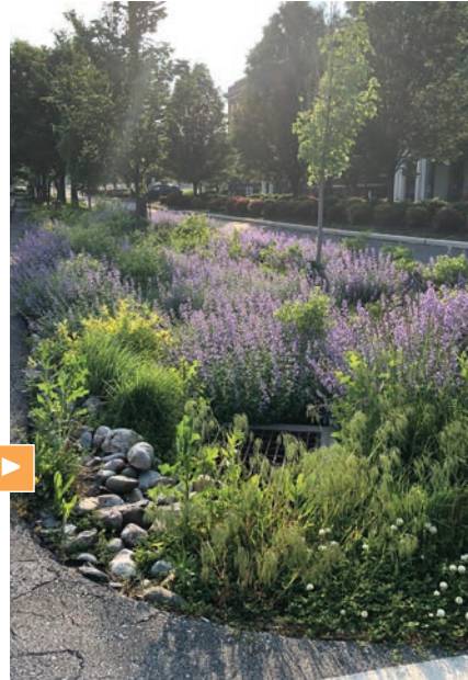
Bioswale between parking lot and roadway in Lancaster City, PA.
