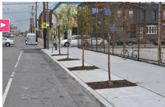
Tree trench on the sidewalk along an urban street. (Photo Credit- "Washington Ave Tree Trench" by Philadelphia Water Department is licensed under CC BY 2.0).
