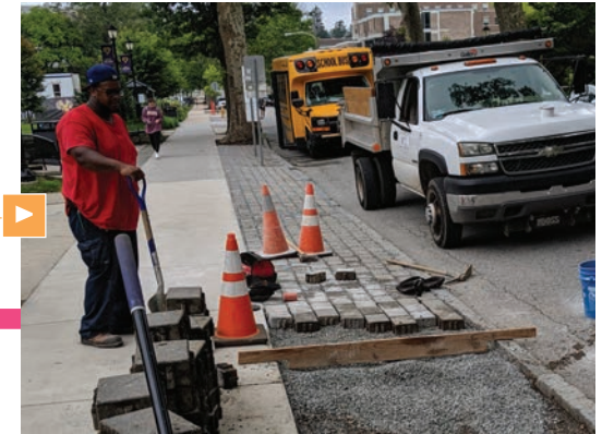
Installing permeable paving at West Chester University, West Chester Borough, PA.
