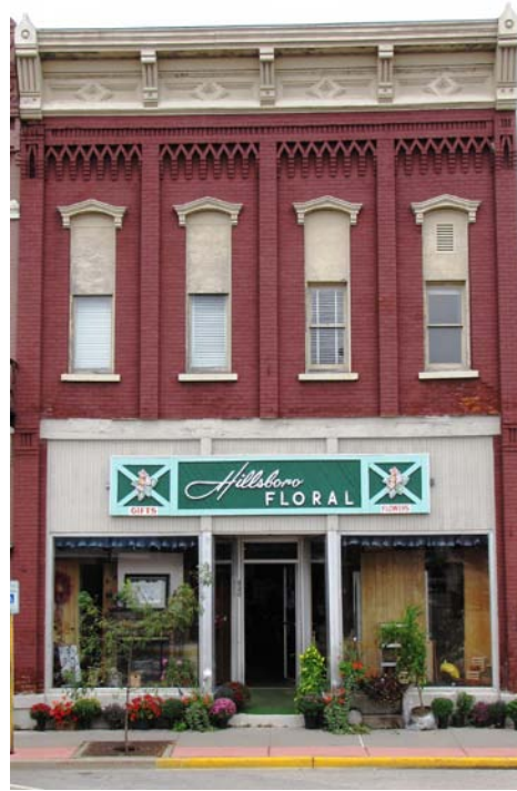
Figure 1.8 – Clearly delineated upper and lower facades.
