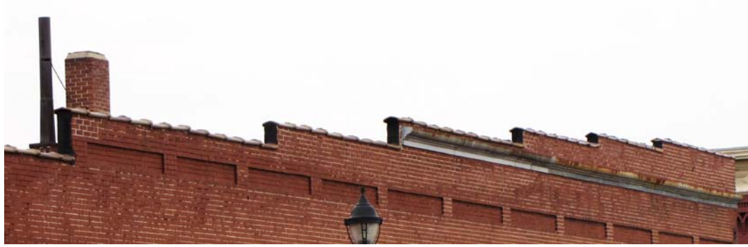
Figure 2.1 – Example of detailed stepped parapets or detailed brick coursing.
