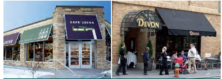
Awnings (left) or canopy structures (right) help define the building entrances and provide visual interest along the street frontage.
