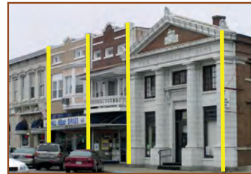
Desired vertically-proportioned buildings.
