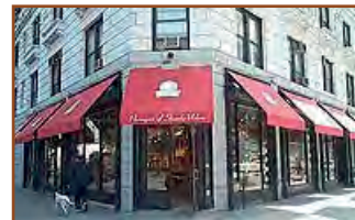
A good example of mounted awnings placed below the horizontal expression line.
