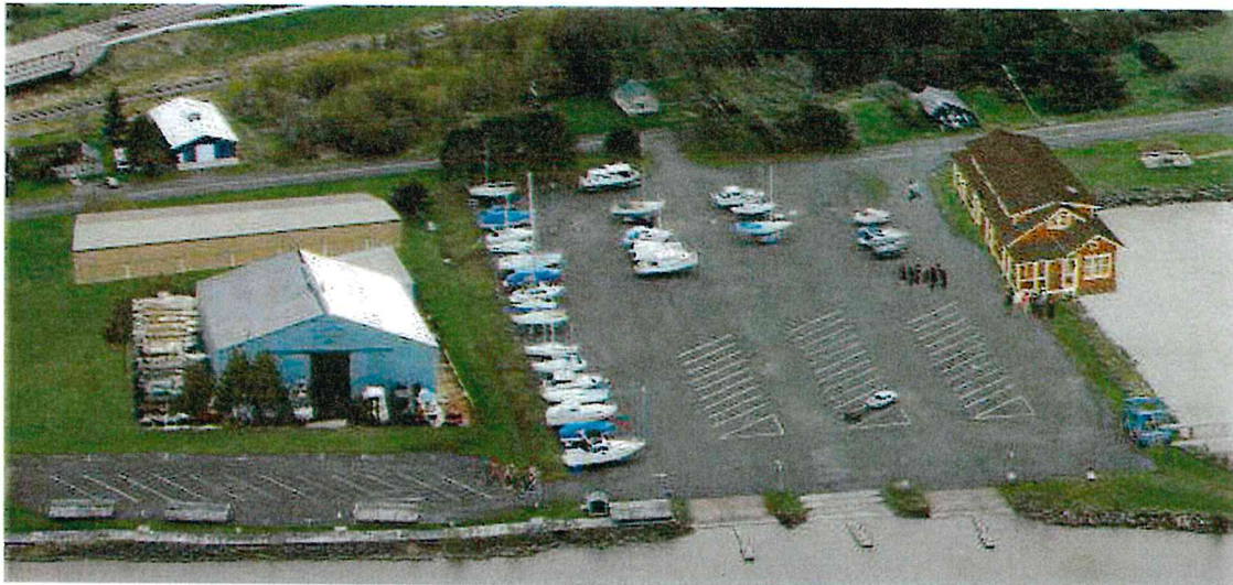
Figure 25 - Existing Condition and Artistic Rendering of Indoor Boat Storage and Boat Club
