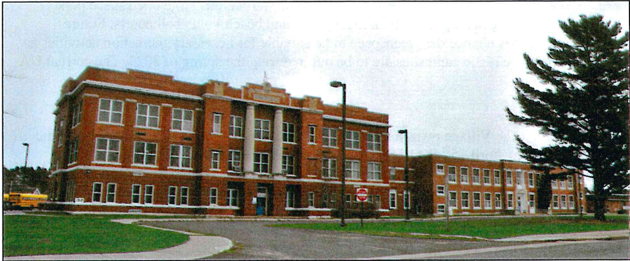
Figure 10: Acquired Ontonagon Elementary School Property
