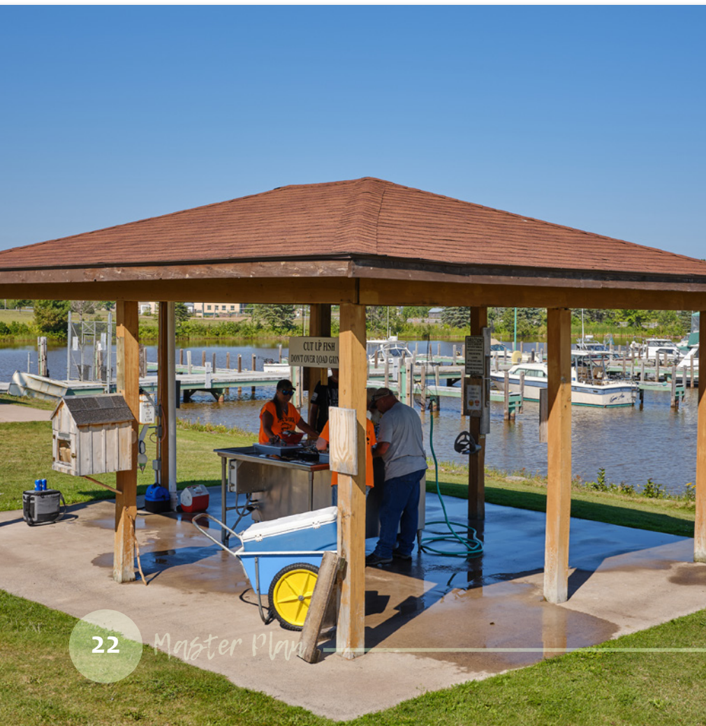
FIGURE 4.4 – FISH CLEANING STATION
