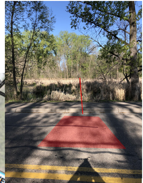
10 x 10 Lining pit in S. Shore Drive
