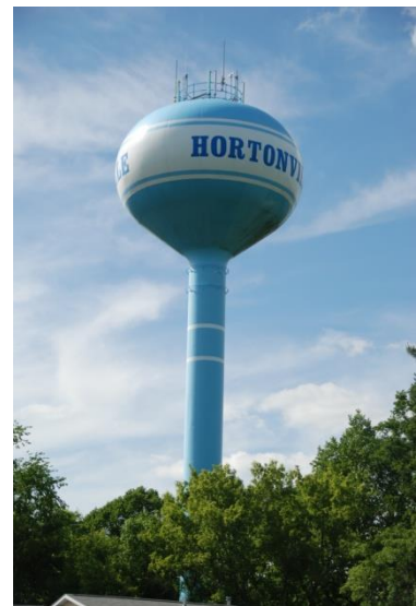
Hortonville Water Tower
