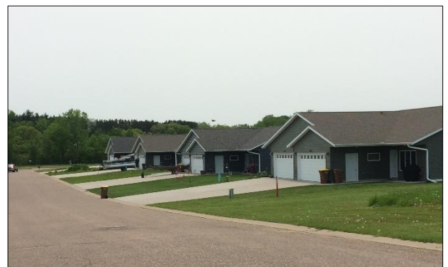
Duplexes on North Creek Lane
