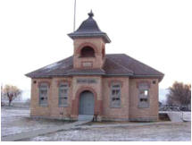
Fairfield School House, 1898
