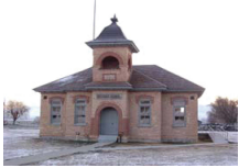
Fairfield School House, 1898
