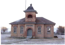
Fairfield School House, 1898
