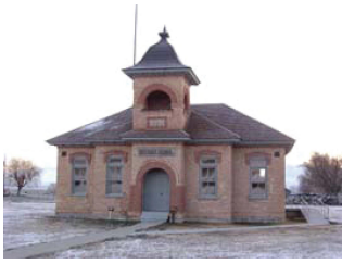
Fairfield School House, 1898
