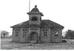
Fairfield School House, 1898
