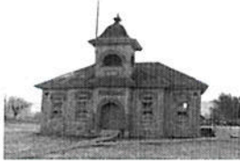
Fairfield School House, 1898
