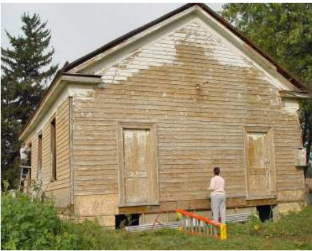
Left: Volunteers spent two weekends working on paint removal in October.
