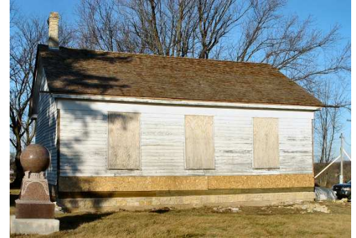
New rim joists and a center beam are now in place and the stone work around the foundation is complete.
