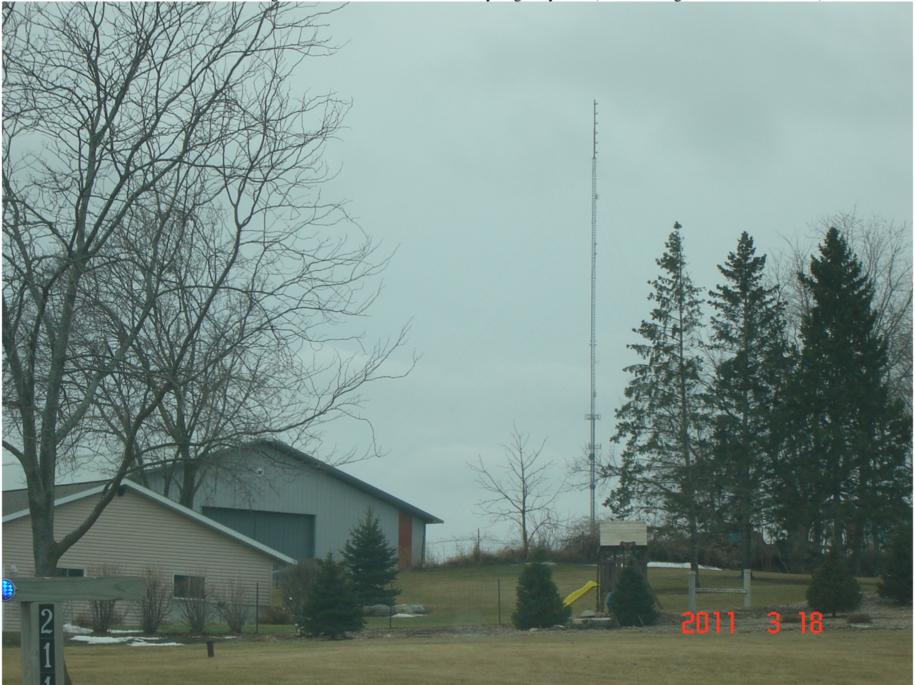
#1: Mid-West Management 499' tower at 1975 County Highway MM (view looking west from CTH MM)
