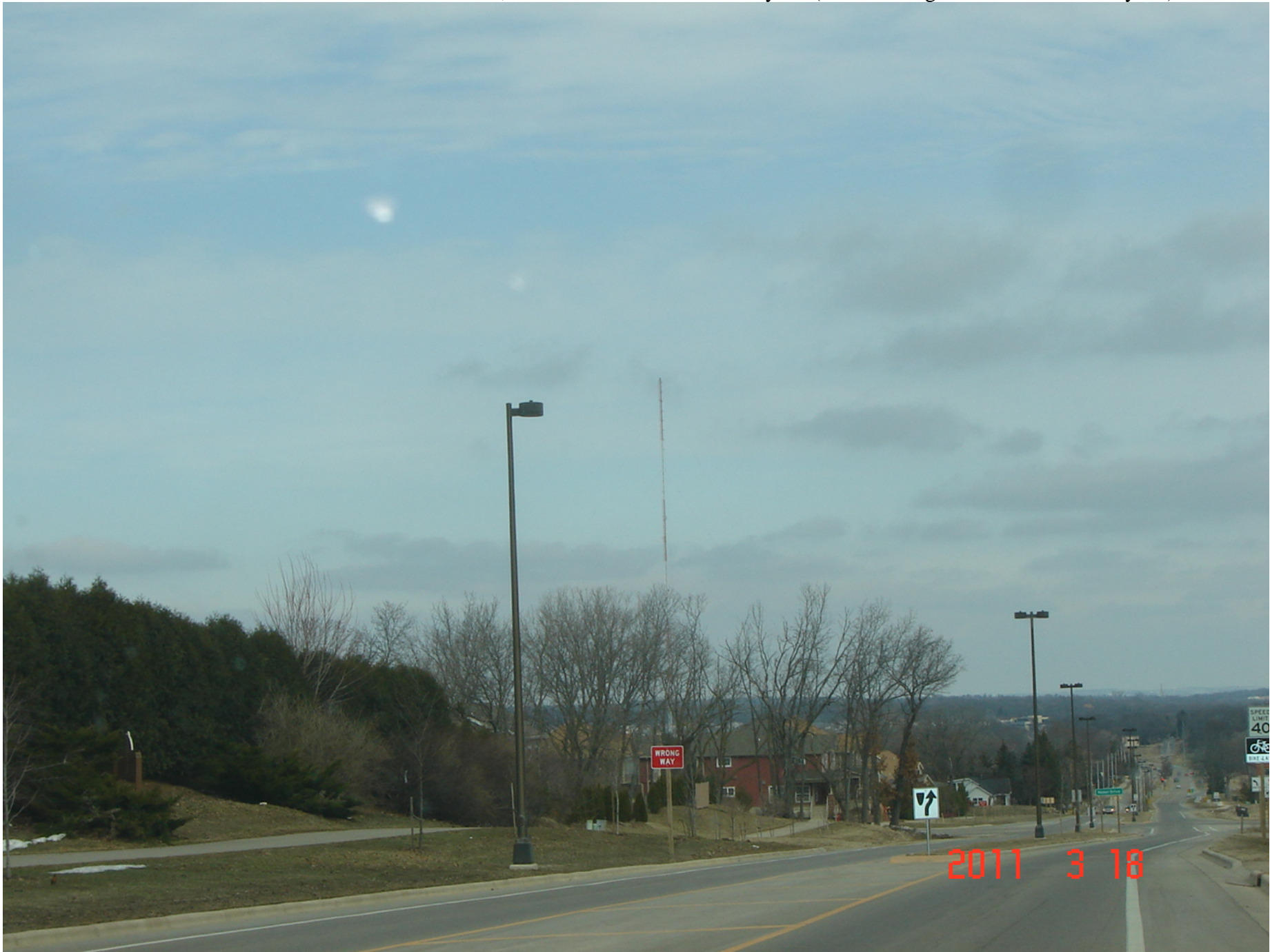
#5: Central Star Communications 433' tower, located at 2651 Fish Hatchery Rd (view looking NW on Fish Hatchery Rd)
