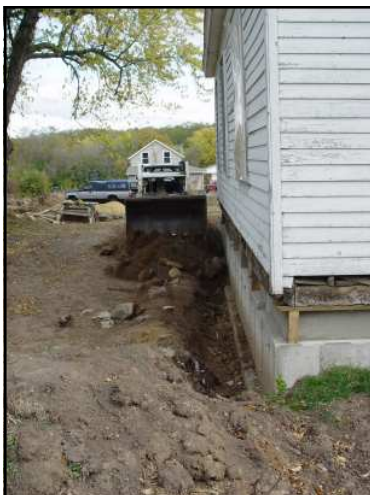
Between August and October of 2005, contractors raised the church, excavated beneath it, and dropped the building onto its new foundation.
