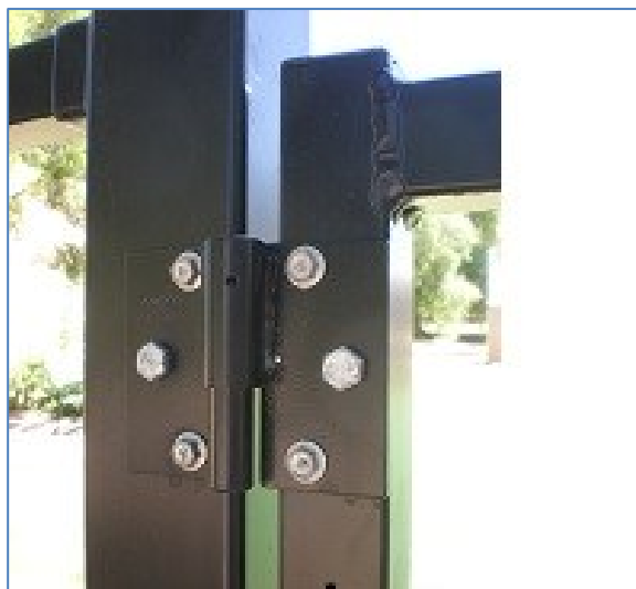
Goliath hinges fitted the gate post and hinge stile of the gate leaf.
