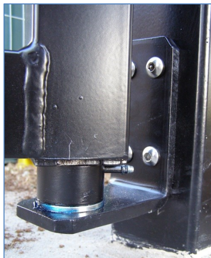
Heavy duty (HD1) tapered roller bearing.
