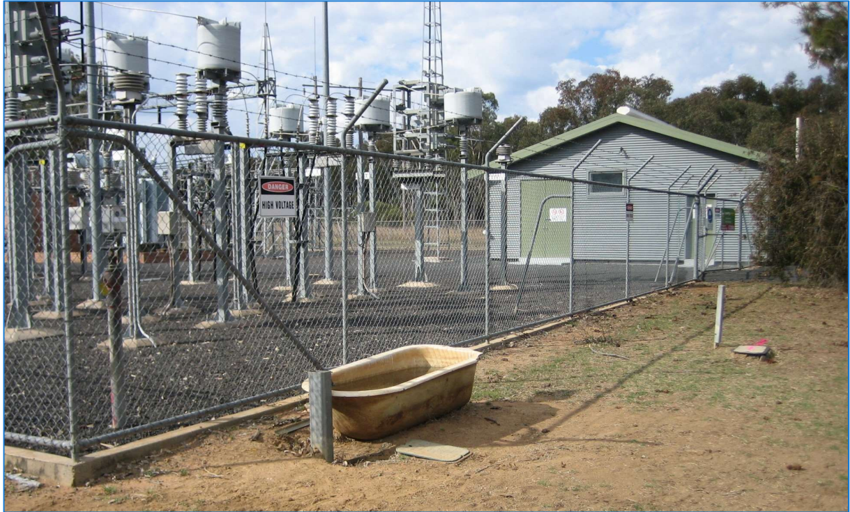
Prior to commencing the security fencing upgrade (Coonabarabran)
