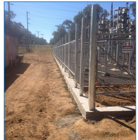
Posts erected and the polyfibre concrete mowstrip placed (Coonabarabran)
