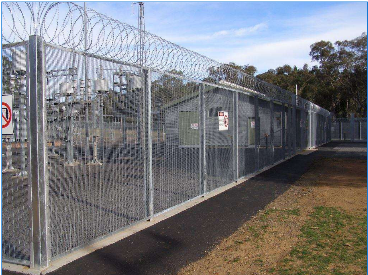
Fencing project complete (Coonabarabran)
