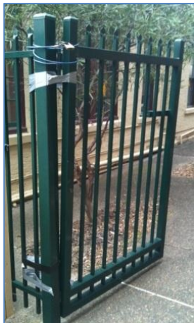
This gate has failed due to the top and bottom hinges seizing and failing.
