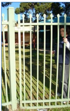
A school teacher holds a gate that had fallen off due to not fit for purpose hinge being used and installed (incorrectly).
