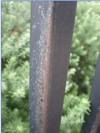
Red rust starting to appear through the powder coating at 3 years.
