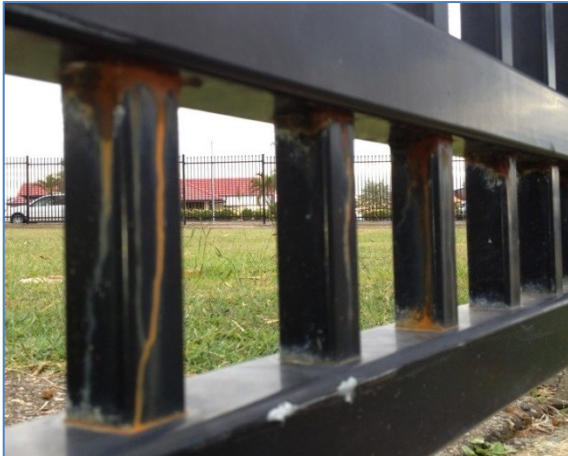
This corrosion suggests the tube may not be galvanised internally
