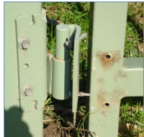
A goliath hinge tek screwed to the gate post and gate stile. The hinge has been installed upside down, it has seized resulting in the teks pulling out of the wall of the gate stile.
