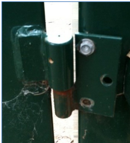
This is light weight Goliath ball bearing hinge that has seized and failed. These hinges are not sealed and cannot be greased. Tek screws have been used installed of a bolt through the post. Two of the three teks have failed.
