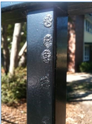
Blistering of the powder coating is a result of poor quality metal surface preparation on an imported panel. Fence installed 18 months.
