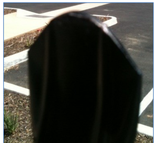
This was a sharp spear picket (on an imported panel) that has been rounded with a grinder to meet the specification. It is already showing signs of corrosion.
