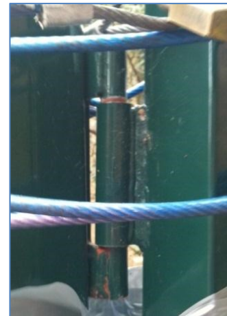
This is a dry top hinge. The pin has corroded, seized and failed.
