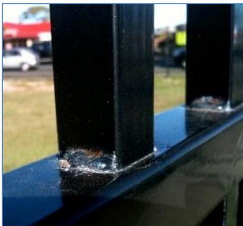
A mild steel or 'black' weld has been used instead of Silicon Bronze which is normally the case with imported panels. The mild steel is hotter than the bronze resulting in damage to the galvanised coating on the tube. In addition the mild steel weld is more prone to corrosion and is a lesser substrate for powder adhesion. This panel had been installed about 12 months.
