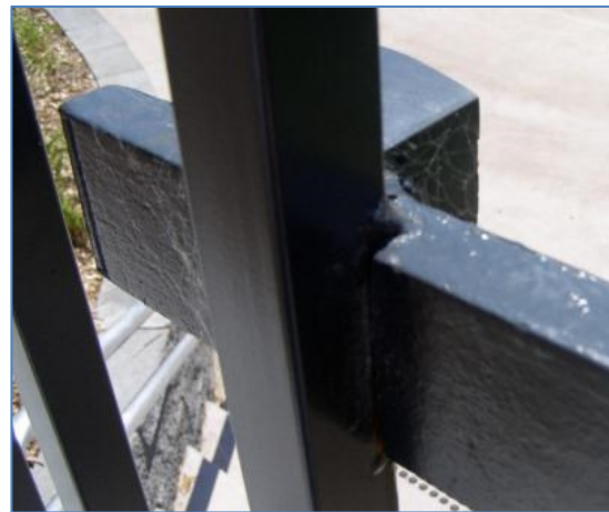
The slide bolt backing plate has been cut onsite to suit the incorrect stile and rail size that has been used.
