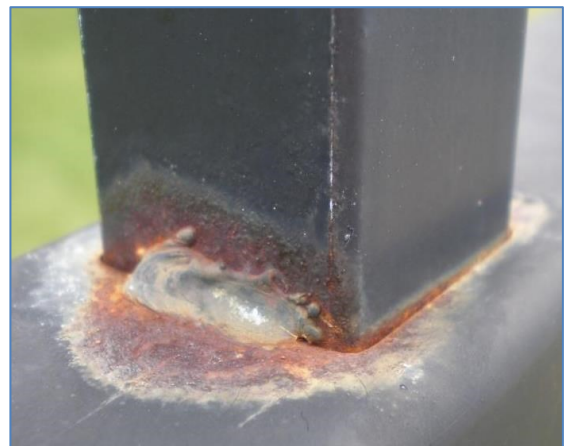
This is an image of the same section of fencing as image at left some 3 years later. Note the severe fading and the aggressive corrosion of the mild steel weld.
