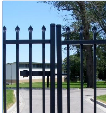
Large double gates swung from Goliath hinges sagging. The gates will soon become inoperable.
