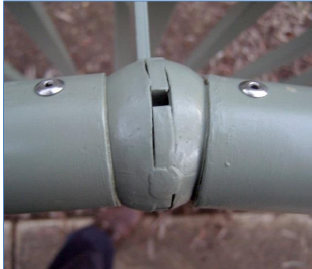
Inward bend: 2 x Ø4.8mm stainless steel rivets in back of Bump Rail picking up the internal Dome Base.
