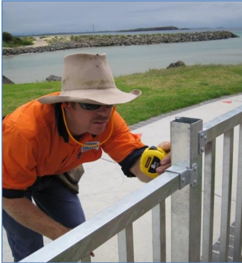
Measuring down from top of post to locate the Standard Bracket and correct height of the Bump Rail.
