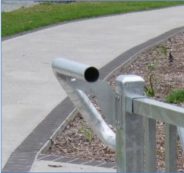
The End Loop (left hand end) secured to Termination Post (P1) and sitting on the Standard Bracket. Ready for swaged end of Rail 1 to be inserted.
