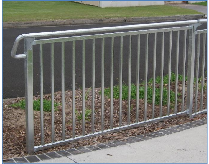
The first piece of swaged bump rail (Rail 1) is connected to the End Loop.
