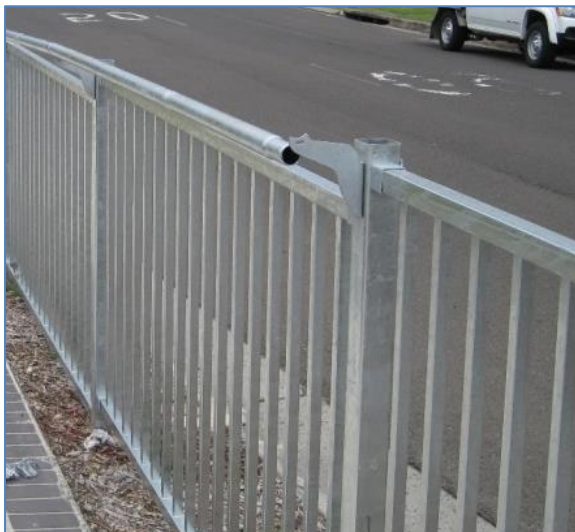
Pieces of Swaged Bump rail being laid out on top of the Standard Bump Rail brackets.
