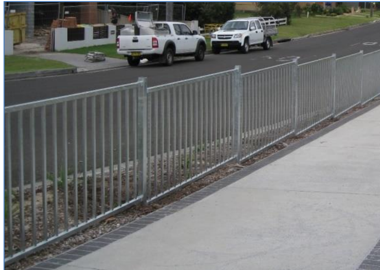
Full barrier assembly. The posts have been set at height to achieve even stepping of the in-fill panels down the gradient and to suit the adjacent riding surface.
