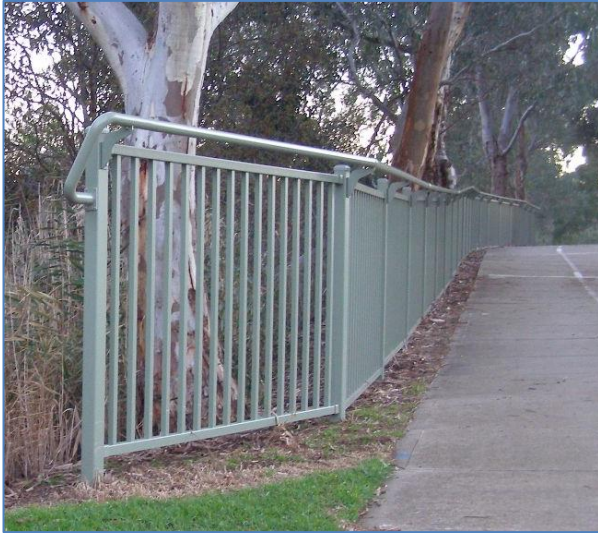
Ideally the first two panels of the run are splayed away to about 1 metre from the edge of the cycleway path.
