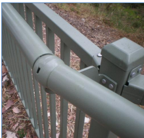
An outward bend with a splayed post
