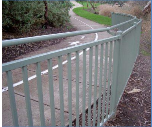
A sweeping bend is divided into short runs of two full panels between changes in direction.
