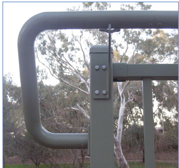
The completed End Loop assembly fixed to the Standard Bracket with a U-clip and rivets and to the first piece of Bump Rail.
