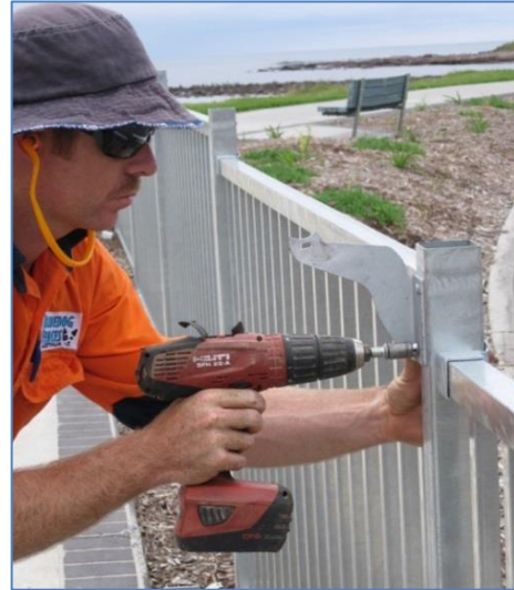
Fixing a Standard Bracket to the post with self drilling tek screws.
