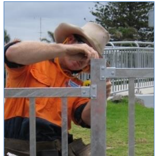
View from backside of the post showing the brackets fixed to the post and stepped to suit the gradient of the path.
