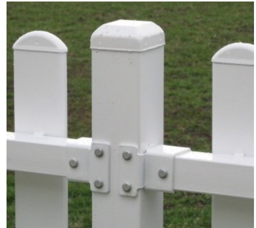
View from outside of the post showing the brackets fixed to the post. The opposing brackets are set at the same height to suit level ground.
