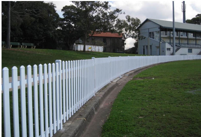
The posts have been set at height to achieve even stepping of the fill panels down the gradient.
