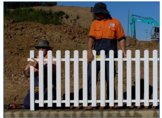
The panel brought to level and the bracket at the other end of the top rail is secured to P2.
