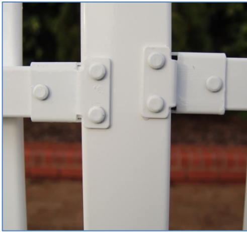
View of the post showing the brackets fixed to the post. These opposing brackets are stepped to allow for the gradient of the terrain.
