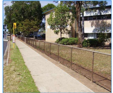
Before: Freemont Elizabeth. The existing 900mm high chainwire fabric fence offers little security.
