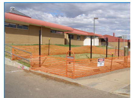
The schools are normally operational and therefore restricting access to the work area is critical.
