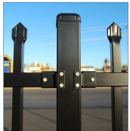
The opposing brackets on the post are set level to suit the level gradient
