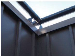
Inset corner installation
