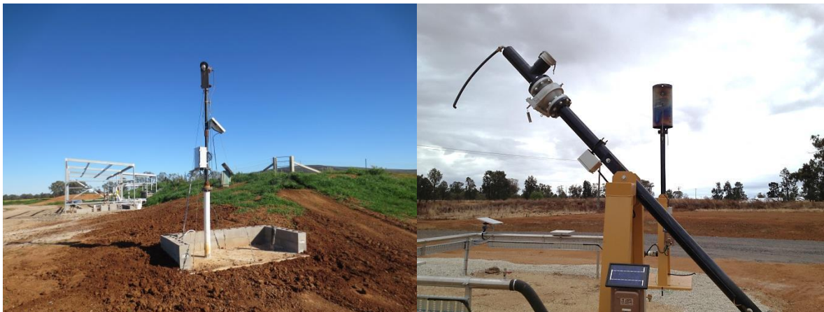
Figure 2.3 Typical on-farm biogas spark-ignition flares in Australia (Photos courtesy of the Pork CRC)
