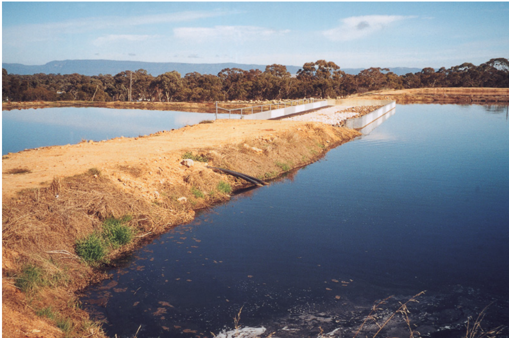
Recently built Anaerobic Pond
