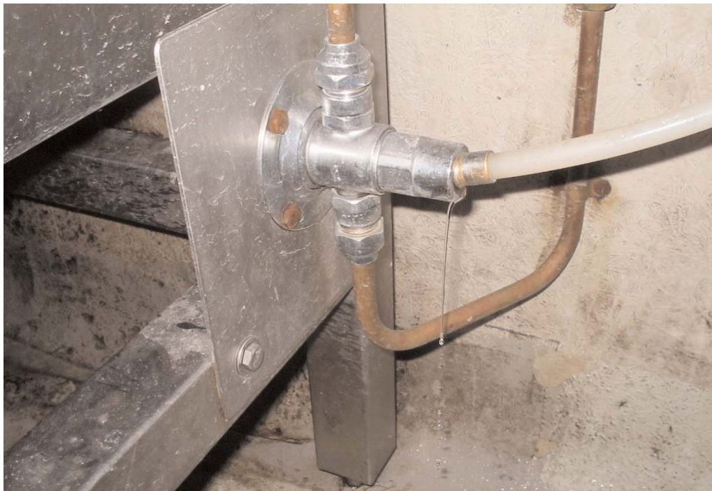
Taking supply water meter readings during non-production hours can highlight any unusual water consumption or leaking pipes.
