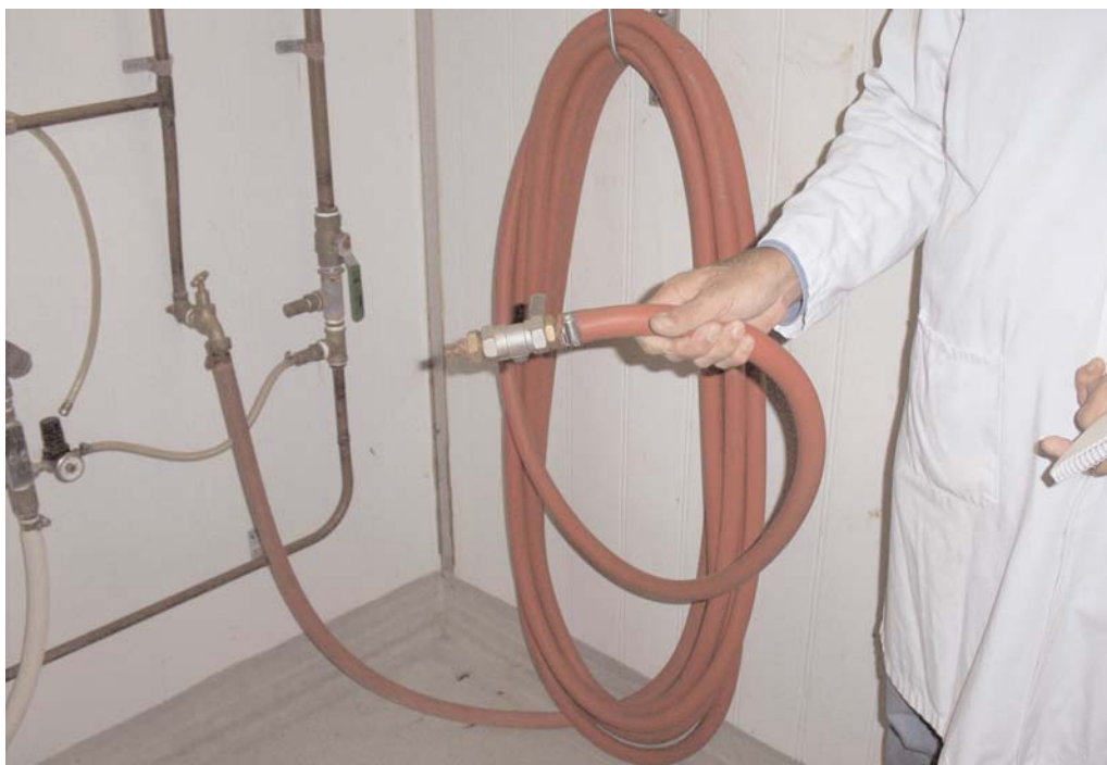
A hose left unattended for a total of an hour a day can waste as much as $1000–$2000/yr.
