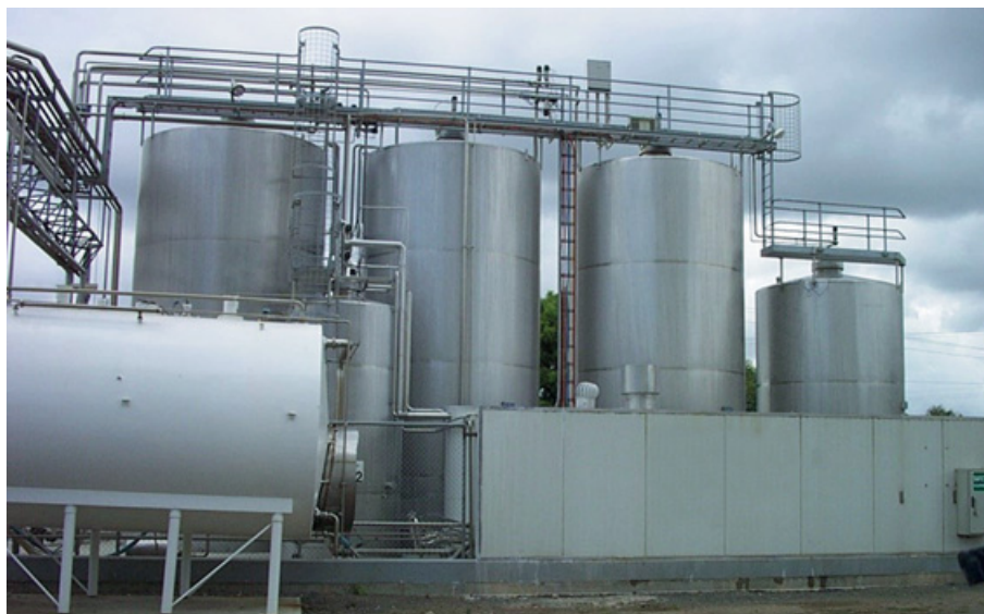
One of the main advantages of CIP systems is that they can recover and recirculate chemicals and rinse water.
