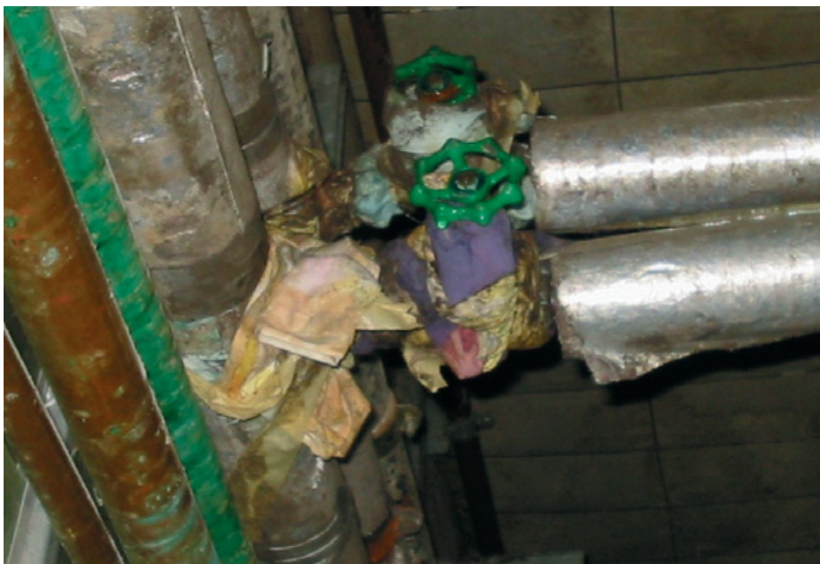
Prevent insulation from deteriorating by eliminating sources of moisture and ensuring that damage is repaired promptly.
