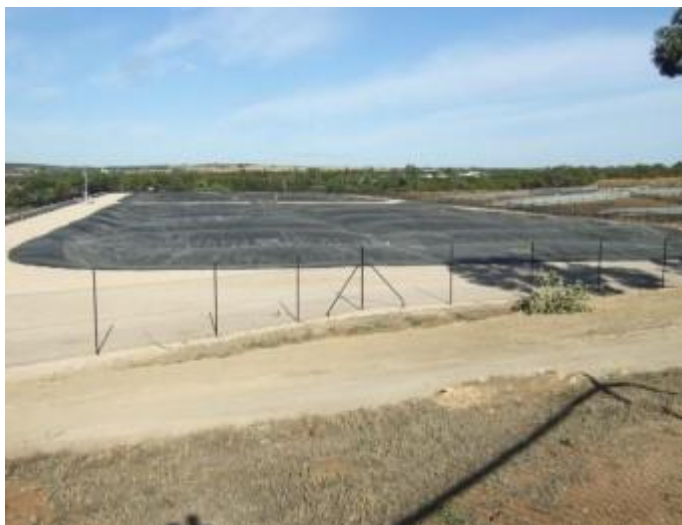
Image 2: Twin 20 ML CALs treating wastewater from a mixed species Australian meat processing facility
