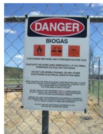
Image 5: Biogas Warning Sign
