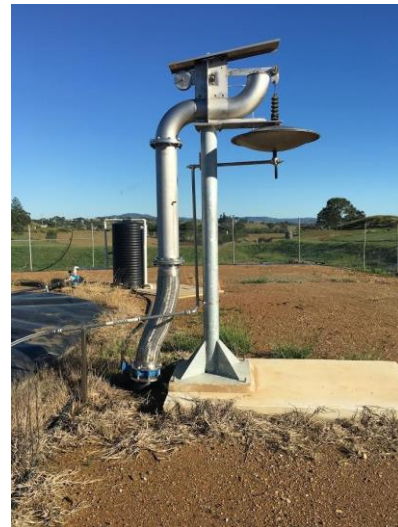
Image 11: Weighted operated flap, Kilcoy Pastoral Company, Kilcoy
