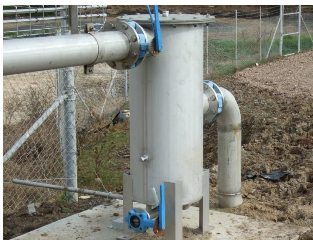
Image 14: Knockout pot in biogas train
