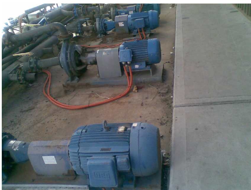
Photo: Variable Speed Drive (VSD) Control of motors offer a more energy efficient alternative to throttling of pumps with variable flow requirements.
