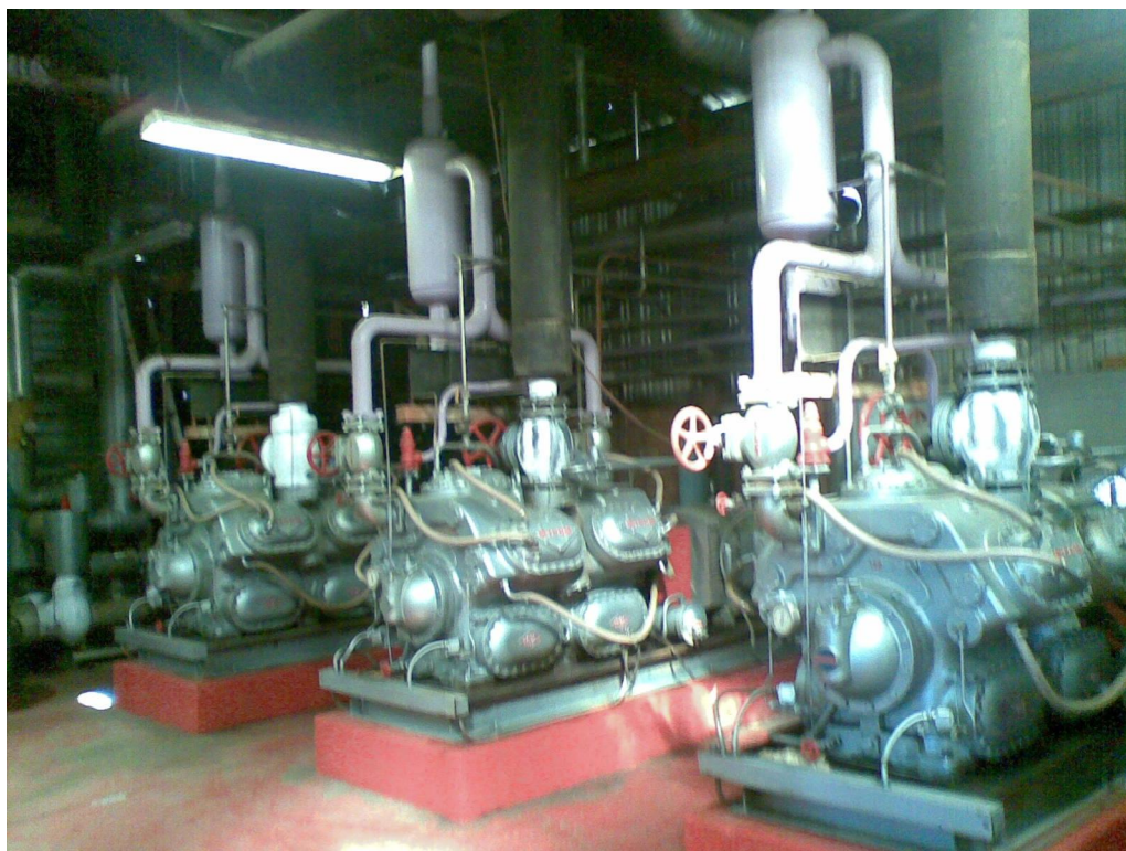
Photo: Existing multi-stage reciprocating compressors can be used as trim compressors to avoid running large screw compressors at low part load
