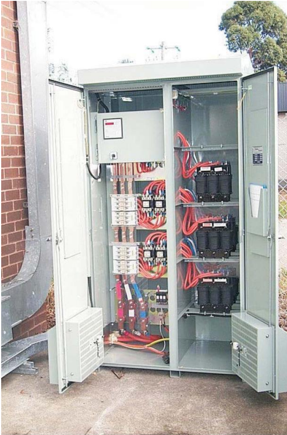
Photo: A 250 KVAR Power Factor Correction System
