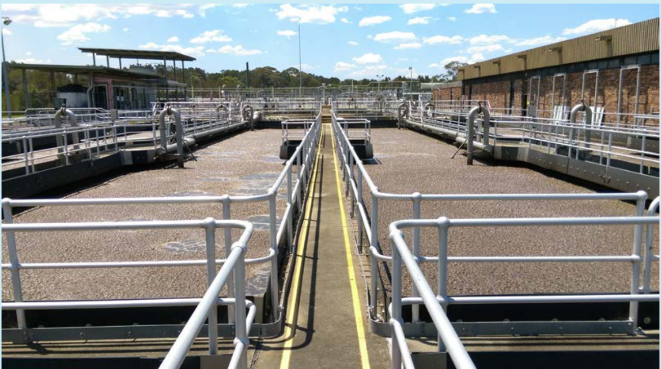
SWWTP bioreactor. Photo: Sydney Water Corporation
