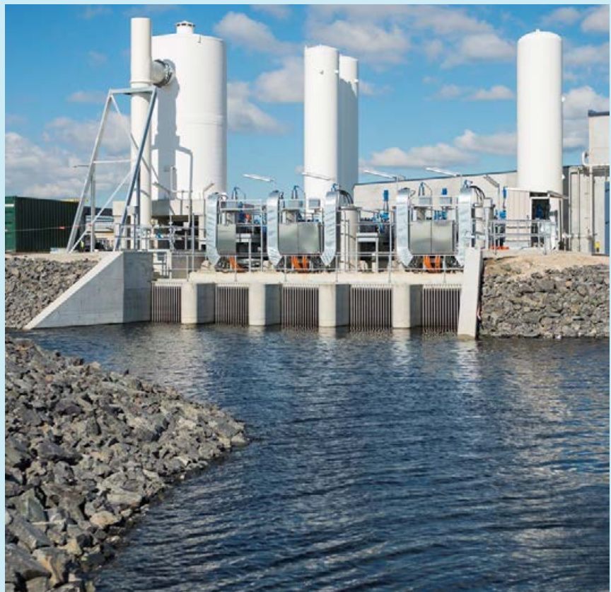
Melbourne Water's Eastern Treatment Plant. Photo: Melbourne Water
