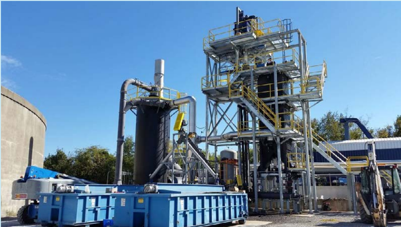
Gasification plant, Lebanon, Tennessee (USA). Photo: Lebanon City Council
