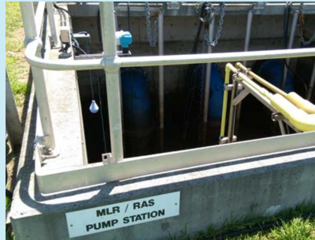
SWWTP RAS tank. Photo: Sydney Water Corporation
