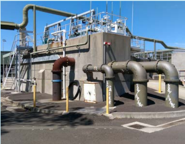
SWWTP Influent piping. Photo: Sydney Water Corporation
