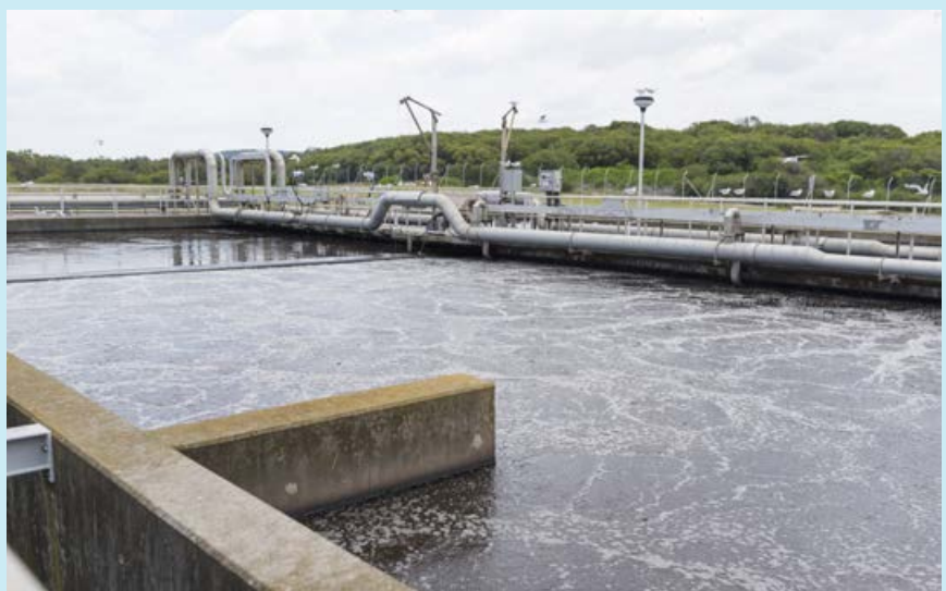
BWWTP aerator tank. Photo: Hunter Water Corporation
