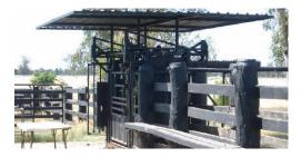
Catwalks should be installed along the forcing pens, race and loading ramp. They should be at about buckle-height, be of sturdy construction and be wide enough to walk along freely and comfortably.
