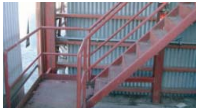
Well constructed stairs with a handrail
