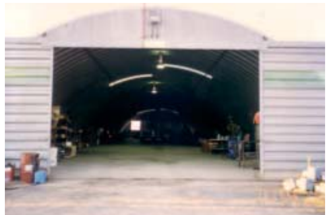
Workshop with unobstructed access
