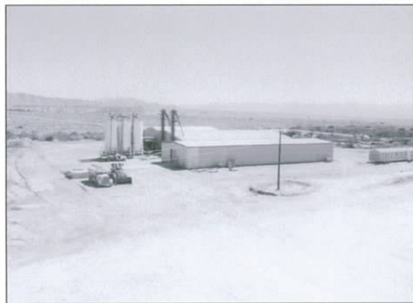
Figure 7. Zeolite processing plant at the Ash Meadows Deposit near the California-Nevada border
