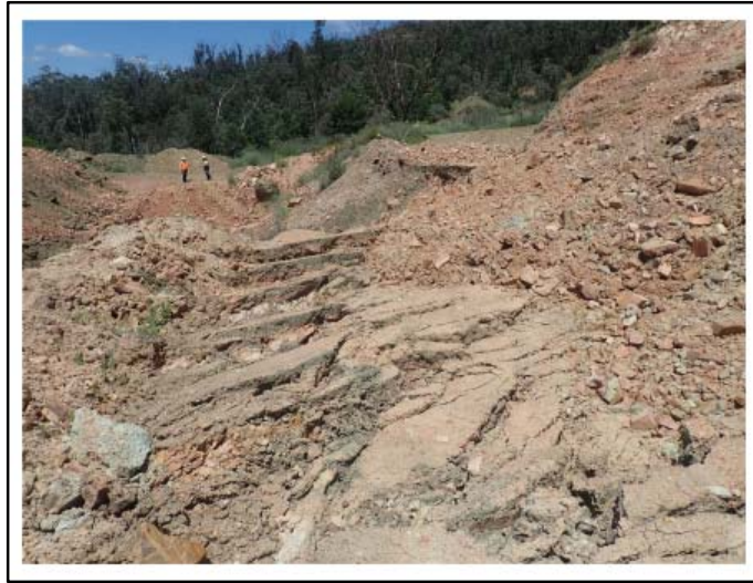
Figure 1 Low wall slip – Eastern end, access road in background and access road deformation
