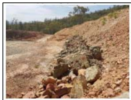
Figure 4 Previously used Boulder Buttress remediation technique
