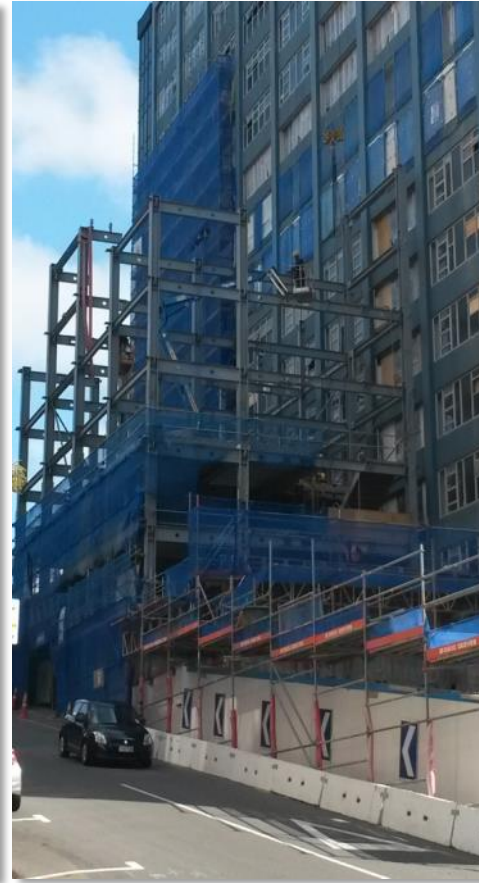
New structure under construction (Mar-15)
