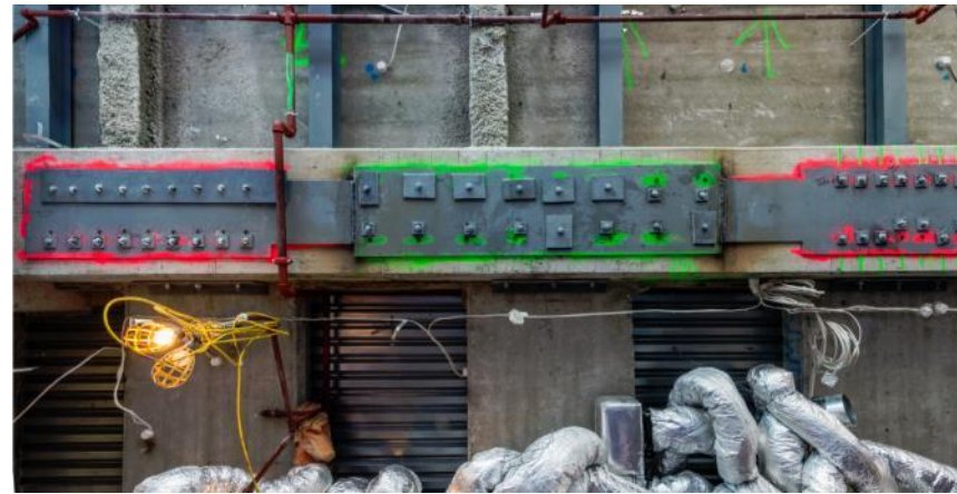
Level 22 wall bracing
