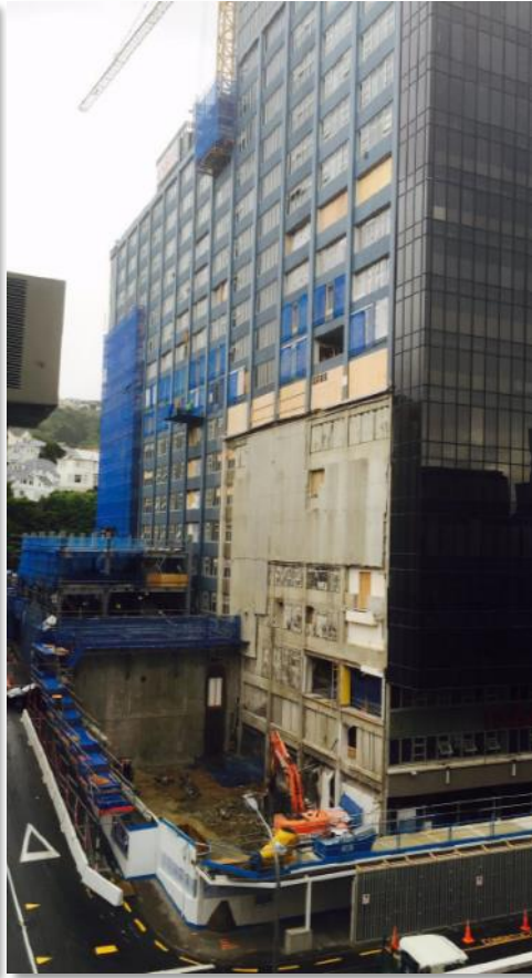
Aurora House demolition
