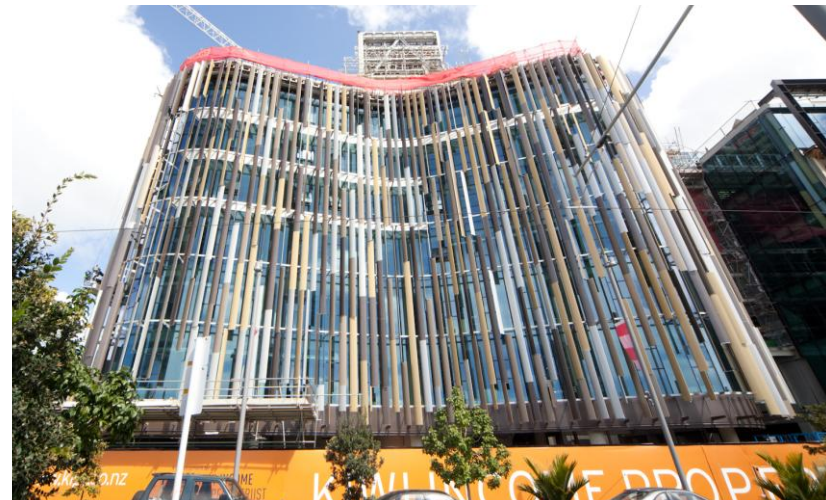
Progress photo October 2012
