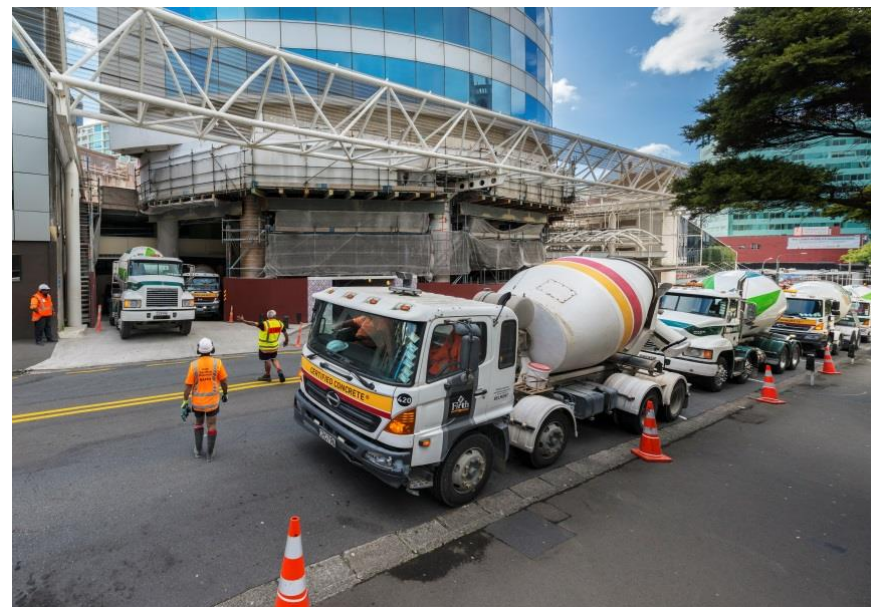
Major foundation concrete pour: 79 trucks, 366 cubic metres
