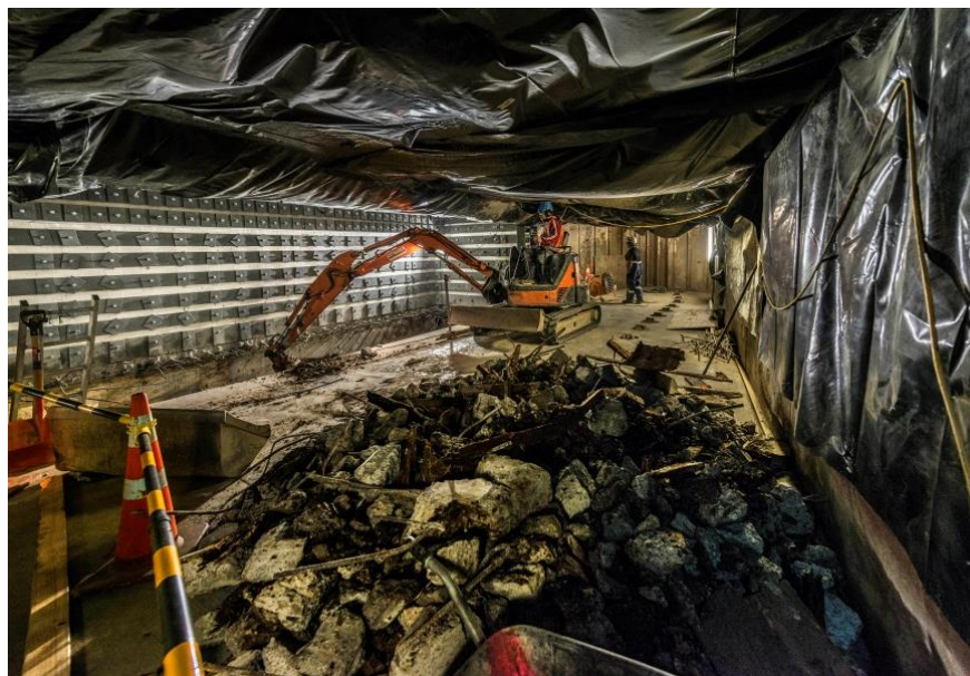
Basement excavation in preparation for new foundation pad
