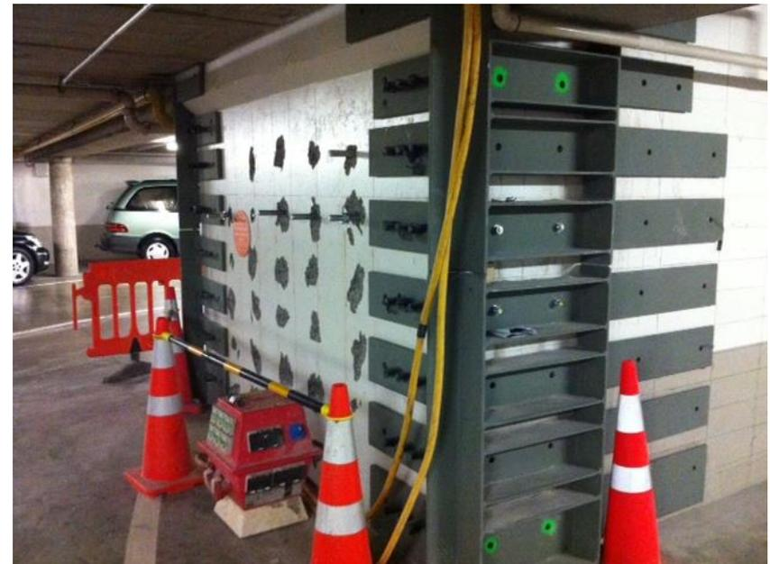
**Shear core strengthened with the addition of 727 tonnes of structural steel, fastened by 15,000 bolts and 8,500 anchors**
