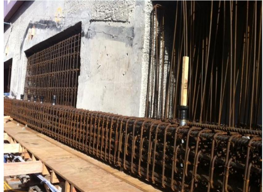
**Transfer beam strength improved with the addition of 74 tonnes of reinforcing steel and 194 cubic metres of concrete**
