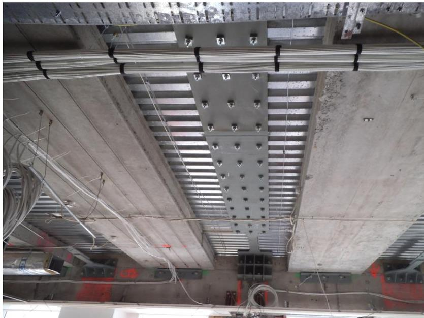
**Tower floors strengthened with 457 tonnes of structural steel fastened by 5,000 bolts, 25,000 anchors and 11,800 metres of post-tensioning strand**
