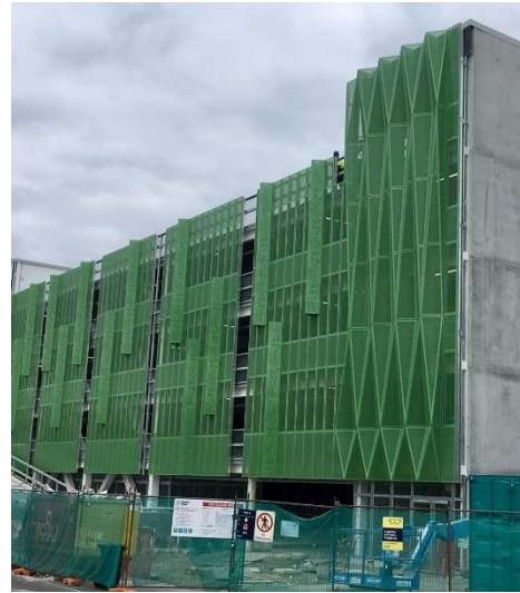
central carpark NEARING COMPLETION
