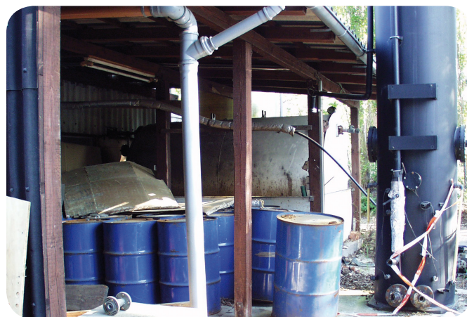
Figure 1: Derelict building with ground pollution at a fur-manufacturing company using chlorinated hydrocarbons for fur-degreasing.
