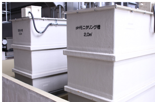
pH monitoring tank (Right) and emergency water tank (Left)
