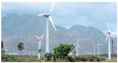
The electrical generators used on wind turbines in sites like Muppandal, produce an output AC of 240 V and a frequency of 50 Hz even when the wind speed is fluctuating. A
