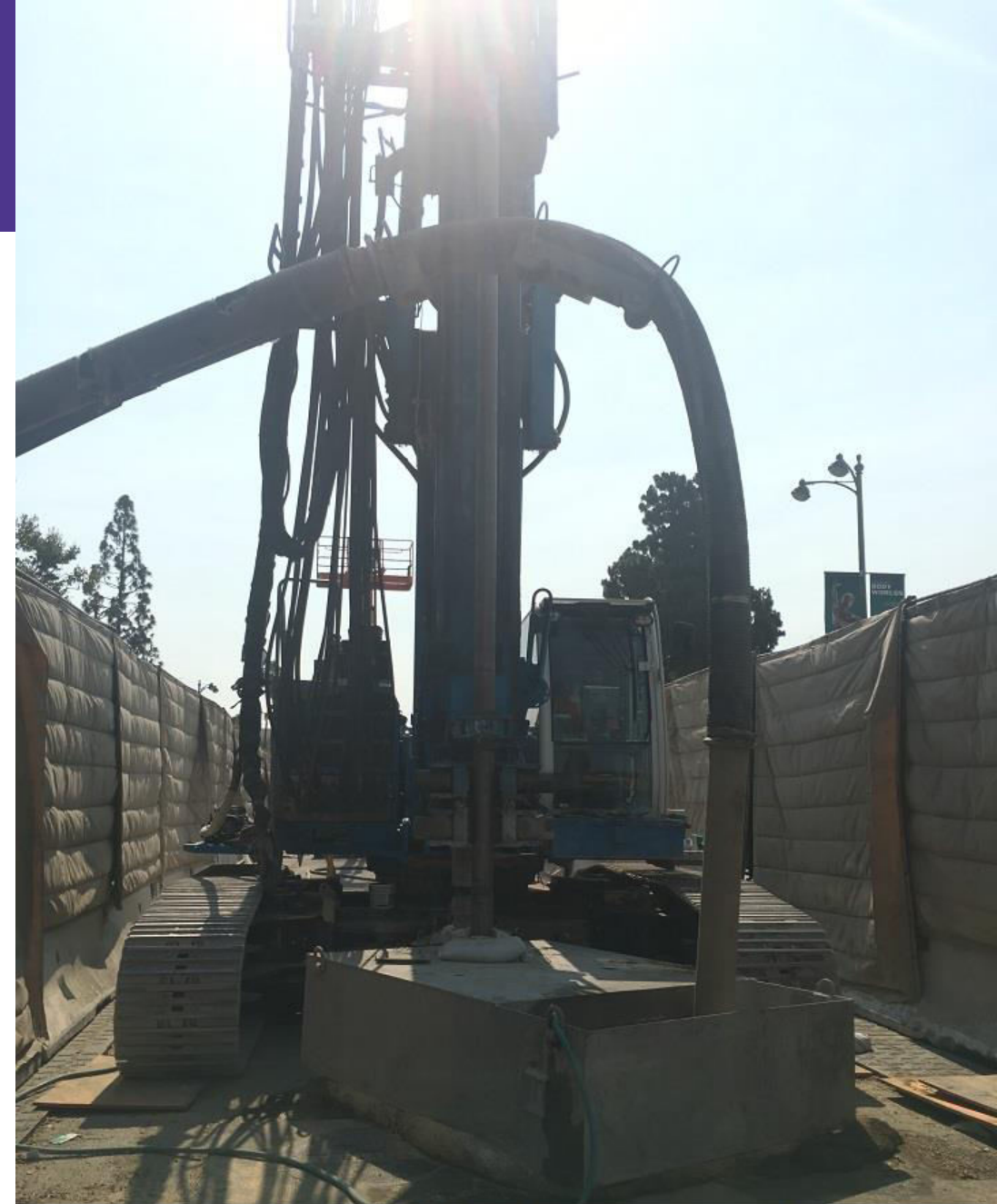
C1045.170712.1000AM Malcolm jet grouting at cross passage 14. Looking E
