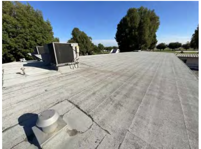
10 - PRIMARY ROOF OVERVIEW
