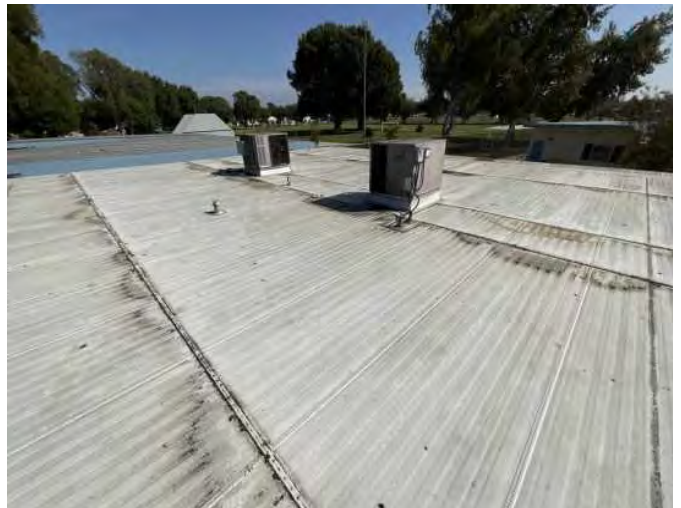
12 - PRIMARY ROOF OVERVIEW
