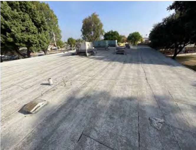
9 - PRIMARY ROOF OVERVIEW
