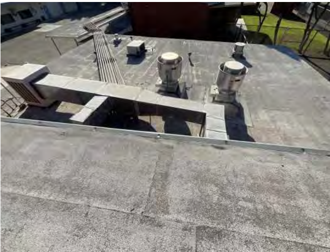
11 - SECONDARY ROOF OVERVIEW
