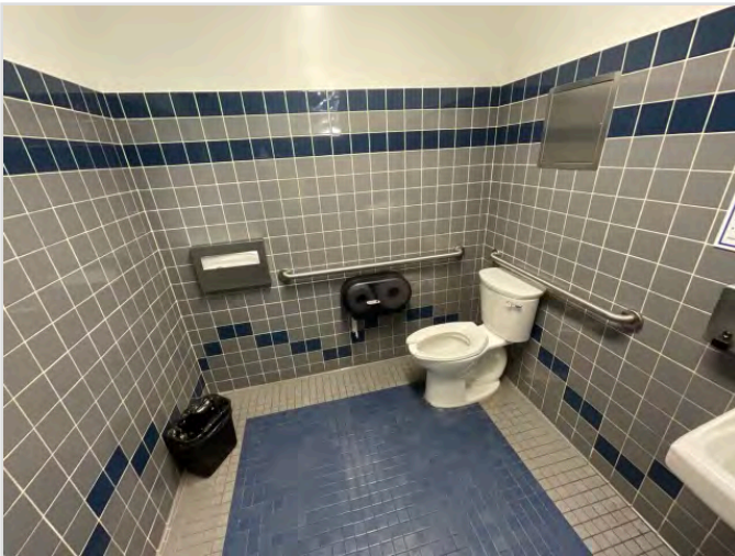
TOILET STALL OVERVIEW
