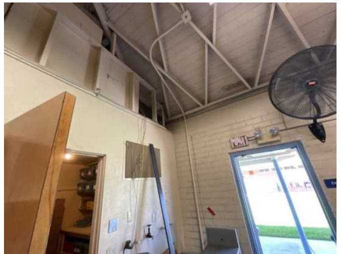
12 - IMC STRUCTURE OVERVIEW
