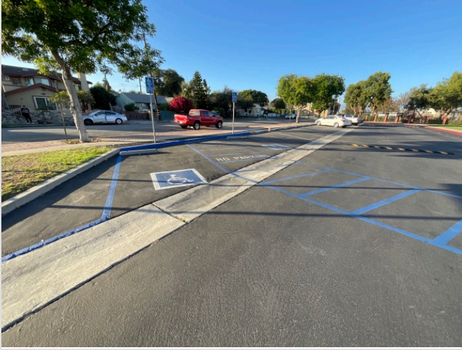
OVERVIEW OF ACCESSIBLE PARKING AREA
