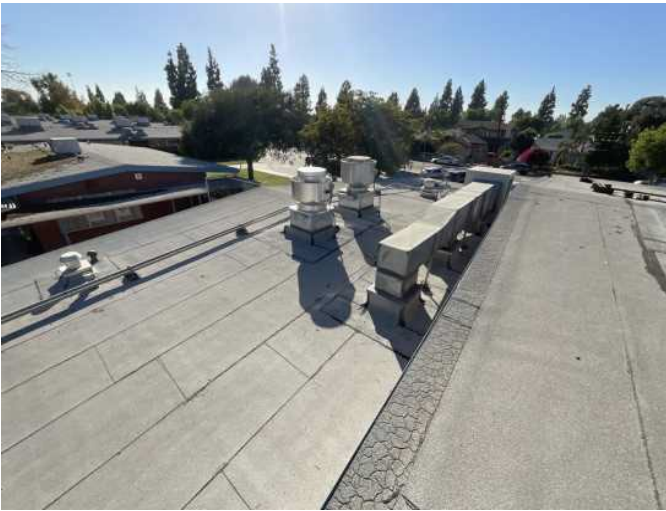
15 - TYPICAL ROOF OVERVIEW
