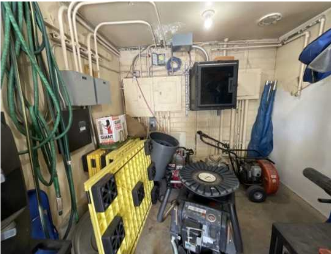
17 - TYPICAL INTERIOR STORAGE ROOM
