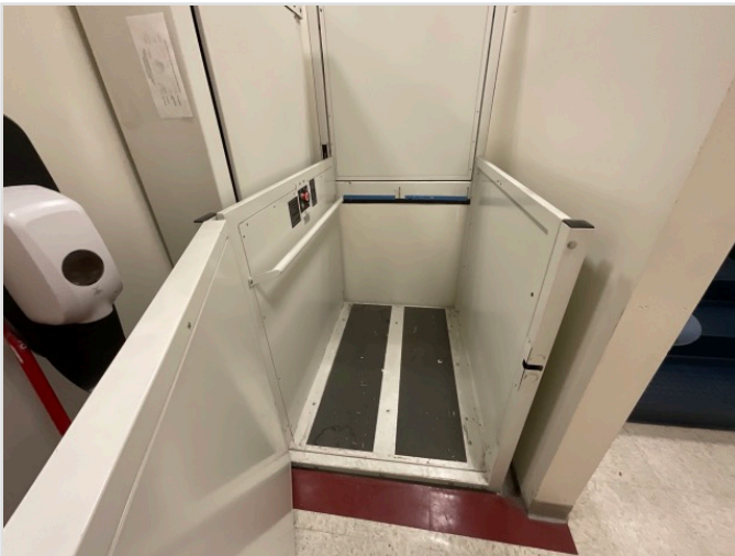
LOBBY LOOKING AT CABS (WITH DOORS OPEN)
