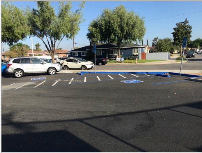
OVERVIEW OF ACCESSIBLE PARKING AREA
