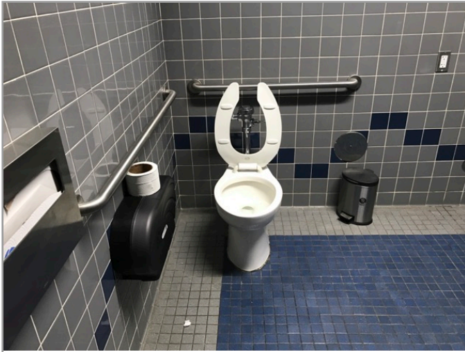
TOILET STALL OVERVIEW
