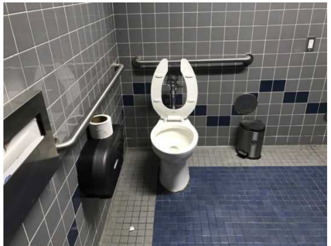
22 - TOILET STALL OVERVIEW
