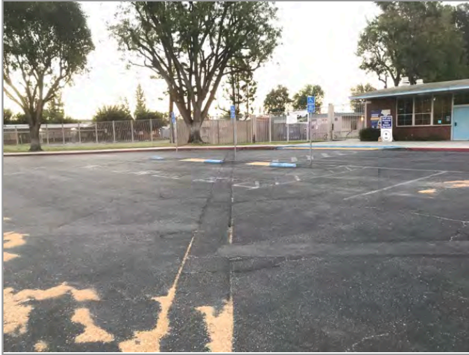
OVERVIEW OF ACCESSIBLE PARKING AREA
