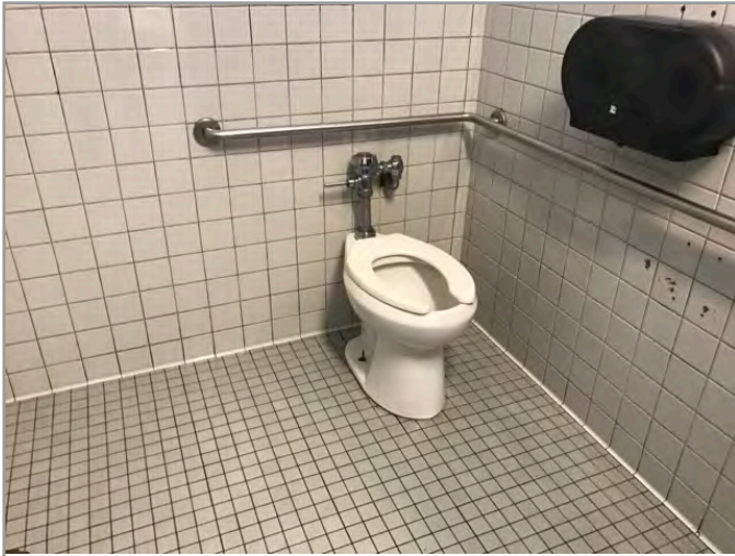
TOILET STALL OVERVIEW
