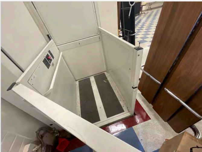
LOBBY LOOKING AT CABS (WITH DOORS OPEN)
