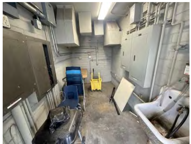
36 - TYPICAL STORAGE ROOM
