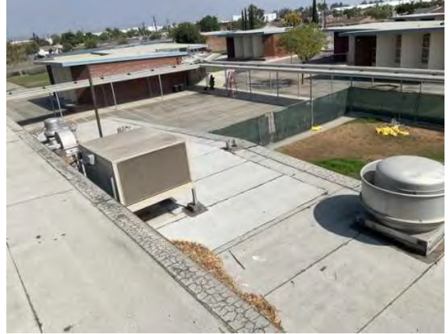
20 - TYPICAL ROOF OVERVIEW
