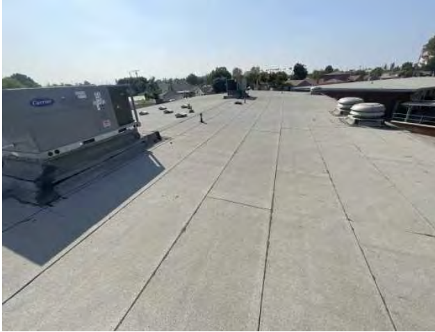
19 - TYPICAL ROOF OVERVIEW
