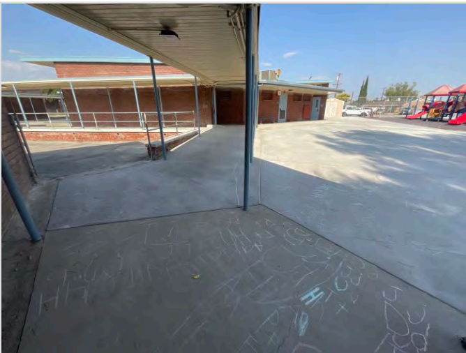
ACCESSIBLE ROUTE TO PLAYGROUND
