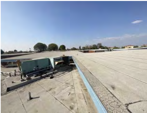
21 - TYPICAL ROOF OVERVIEW
