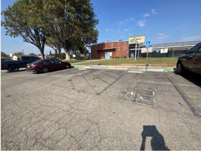
OVERVIEW OF ACCESSIBLE PARKING AREA
