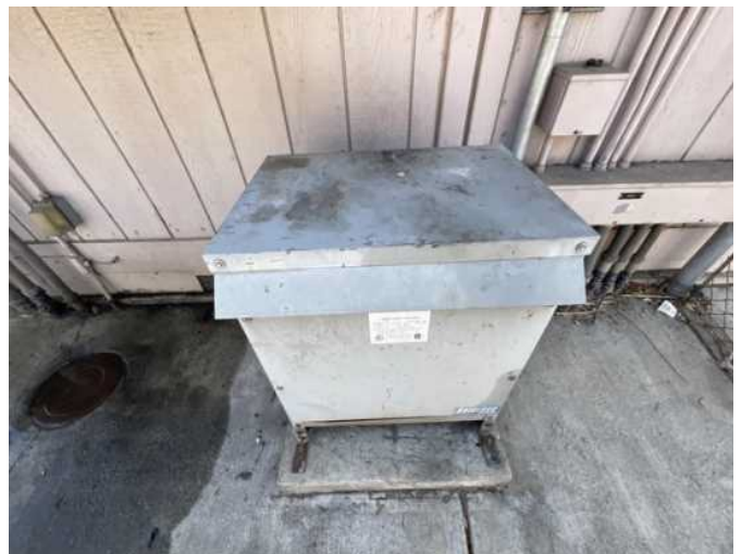
18 - SECONDARY TRANSFORMER
